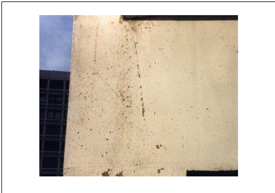
Figure 3(b) Cracking within an external beam-column joint - photograph
